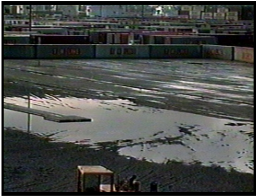
Port of LA CRAM construction site, Jan. 18, 1993, after 11 days of rainfall.
