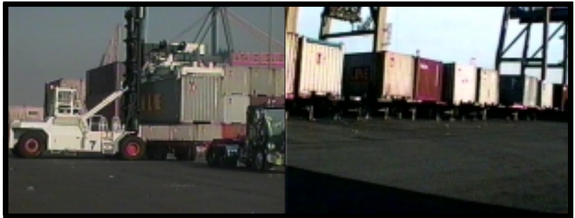
CRAM Pavement at Port of Los Angeles, Berths 127 - 131 Inter-modal yard. The facility is used for loaded container stacking by top-loader and loaded chassis parking.
