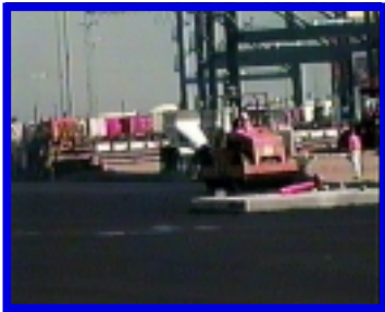
CRAM Pavement; Port of Los Angeles, Berths 127 - 131, Base Asphalt Construction, Utilizing a 6 percent Bitumen Content
